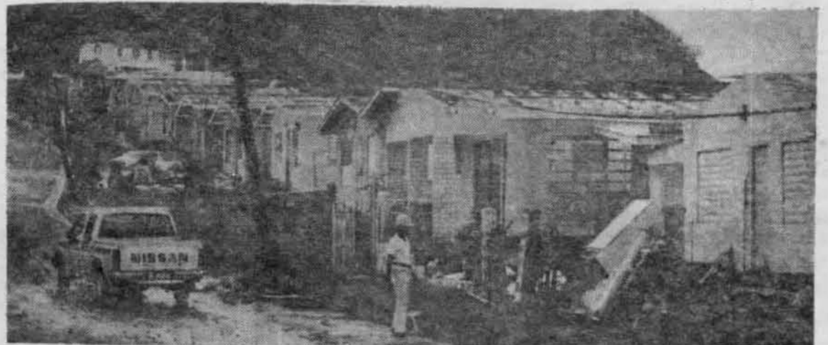
More than 50 per cent of the low-income houses put down in St. Kitts by the Simmonds government had their roofs ripped off by Hurricane Hugo. Photo above shows low-income houses at Conaree left without roofs.
